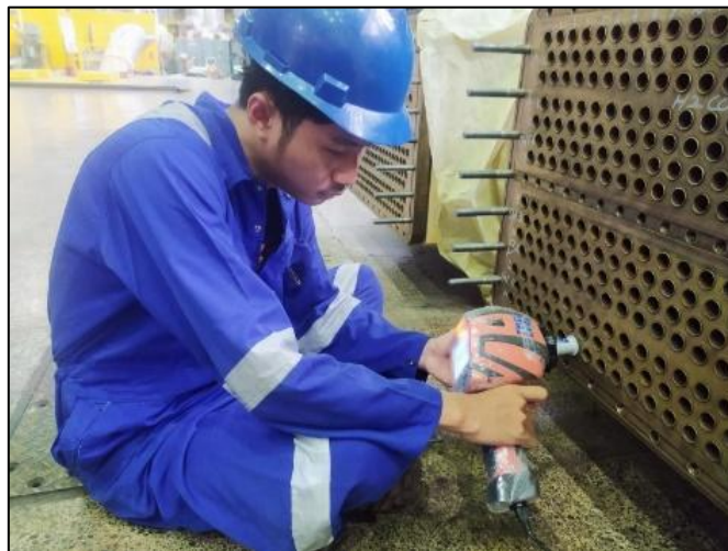
Gambar 4. Proses Inspeksi Tubes H 2 Cooler
