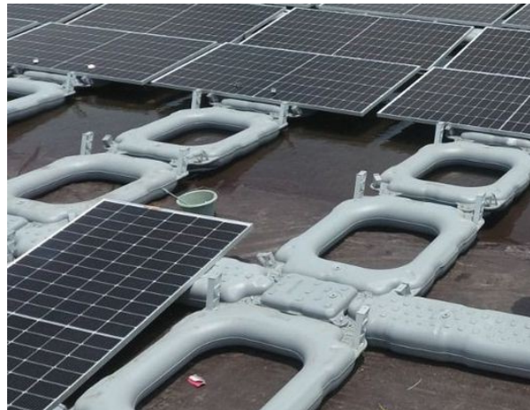
Figure 9. Floater Design for Floating Solar Panels.
