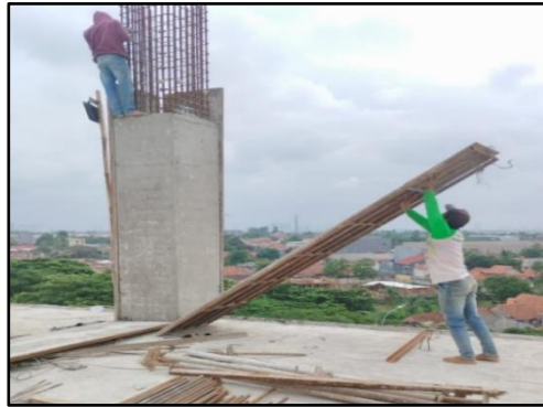
Figure 10. Disassembly Formwork Column
