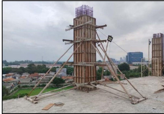
Picture 7. Installation Formwork Column
