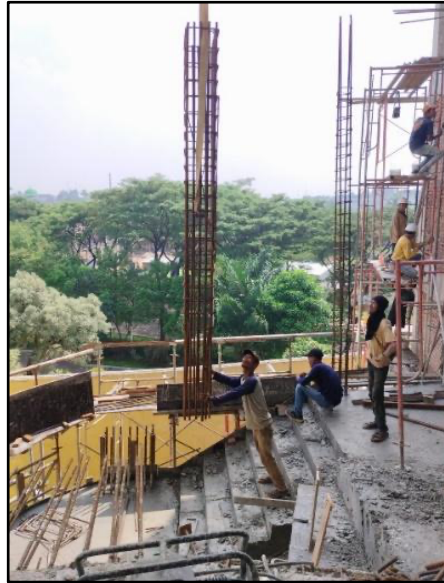
Figure 5. Installation of Column Reinforcement
