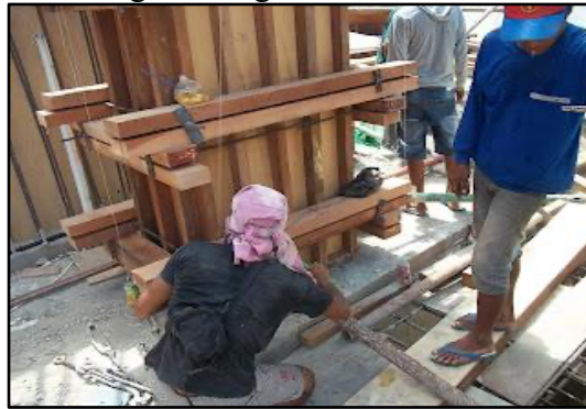
Figure 8. Checking Verticality Bekisting
