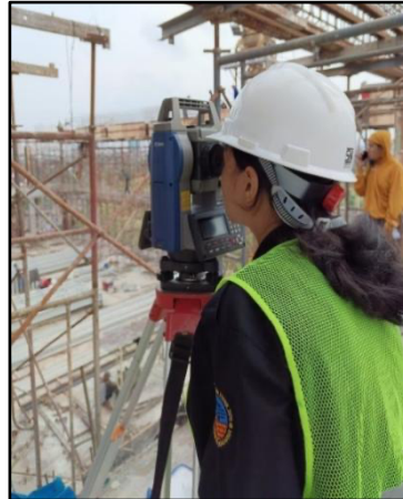
Figure 3. Marking As Column
