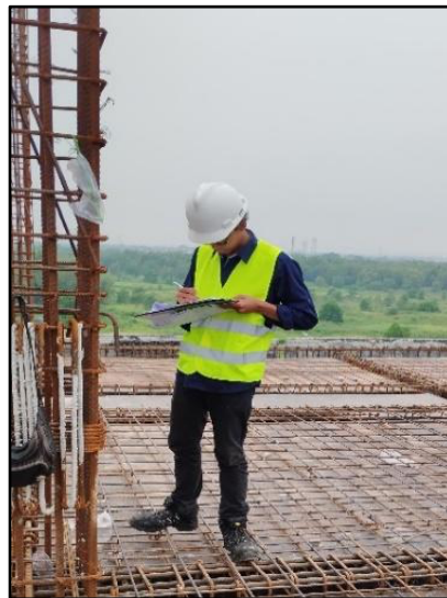
Figure 6. Checking Column Reinforcement
