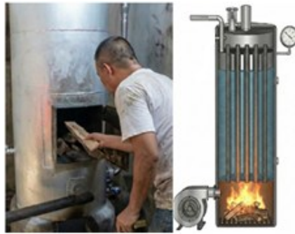
Figure 1. Working Scheme of a Vertical Wood-Fired Boiler
